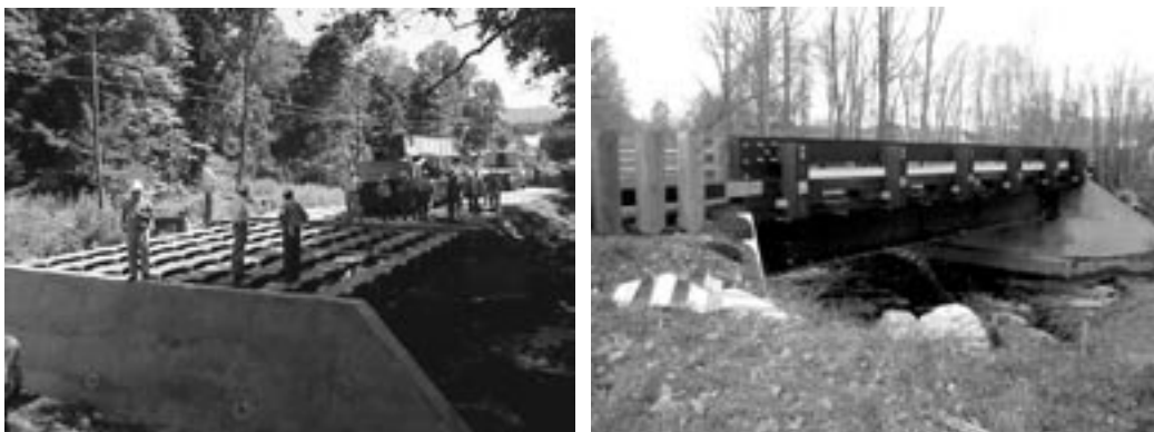
Figure 32. Route 601 Bridge Superstructure
