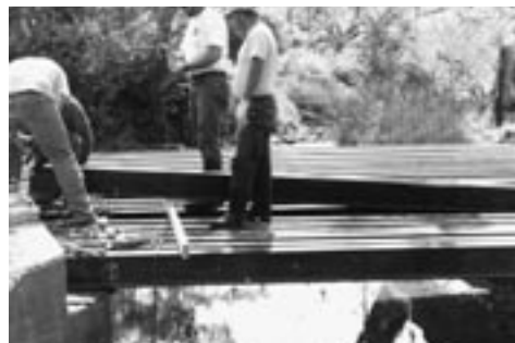
Figure 31. Installation of the Tom's Creek Bridge.
